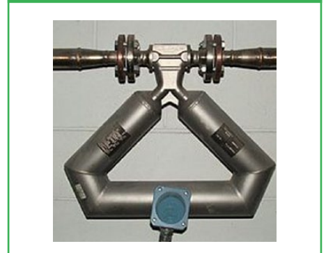
Figure 7. Coriolis flow meter
